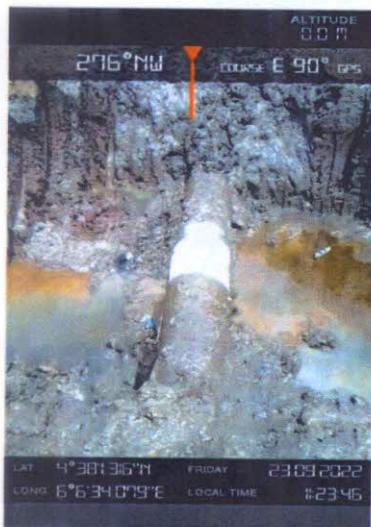
FIG 2-3: Incident Facility repaired and Aqua wrapped
