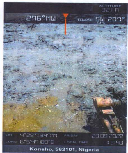
FIG 4: Backfilled Incident Point
