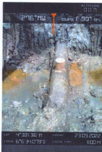
FIG 2-3: Incident Facility repaired and Aqua wrapped
